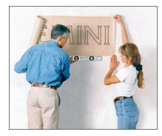
2. Tape one edge of the template to the installation surface with masking tape and unroll it. Level the template and tape the entire pattern securely to the installation surface.
